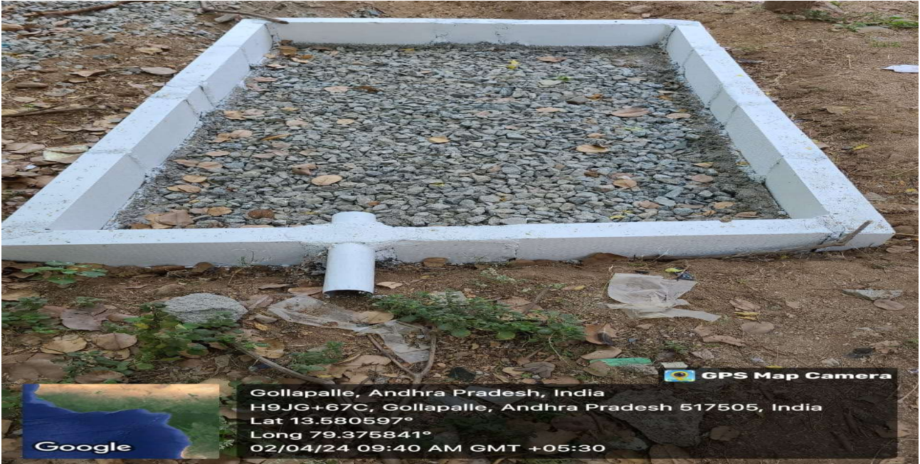
Rain Water Harvesting Pit – 1
