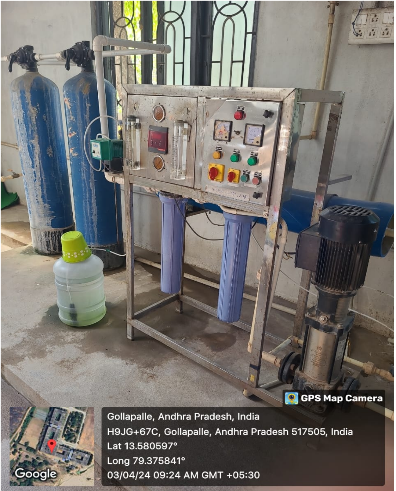
Reverse Osmosis (RO) System (500 Liters per Hour Capacity)
