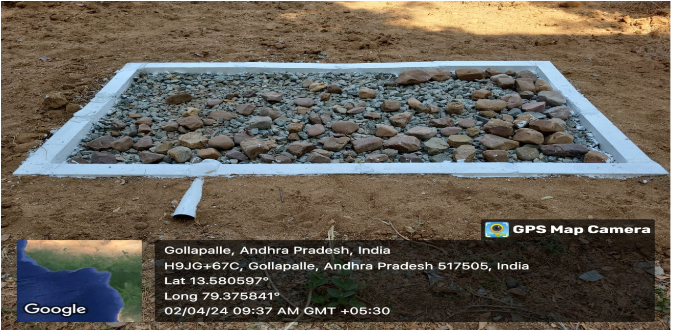
Rain Water Harvesting Pit – 3
