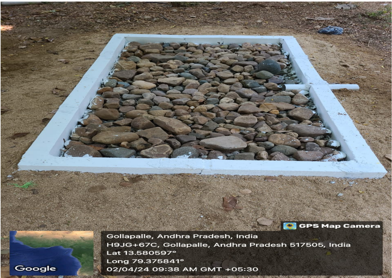
Rain Water Harvesting Pit – 4
