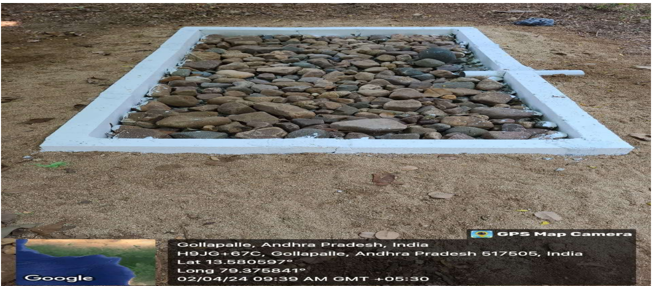
Rain Water Harvesting Pit – 2
